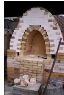
A downdraft, catenary arch style kiln was used for efficiency and ease of construction.
